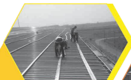
ROOF REPLACEMENT/ ROOFING SHEETS
